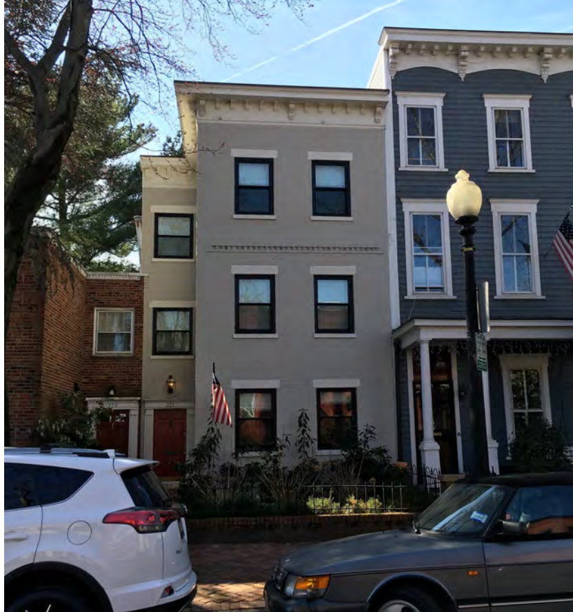
EXISTING FRONT FAÇADE 221 10 TH STREET SE
