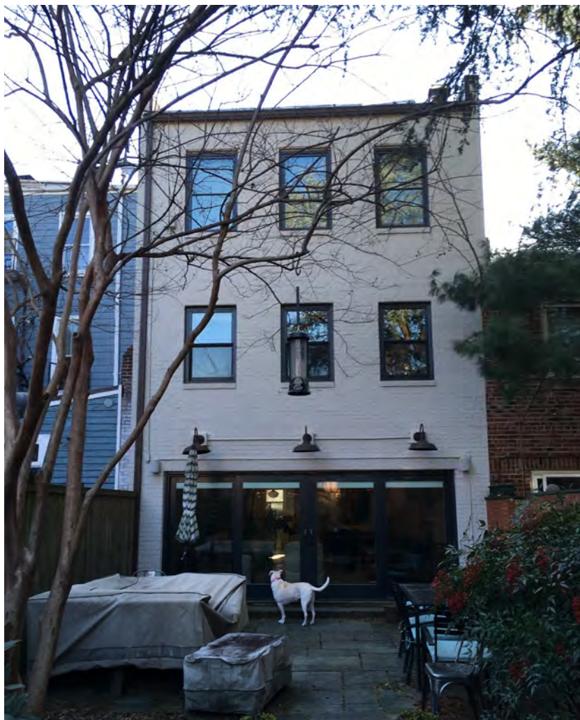
EXISTING REAR FAÇADE 221 10 TH STREET SE
